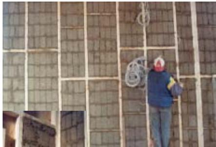
Wood frame walls filled in by clay bricks
