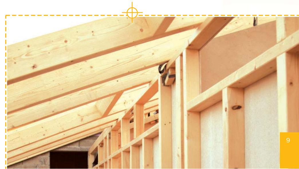
**Wood frame construction in combination with clay**
